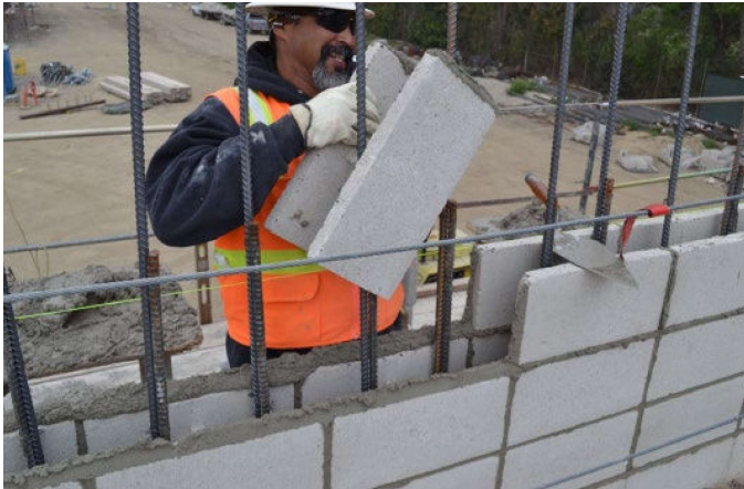
FIGURE 6—Installation of Open-End Units
