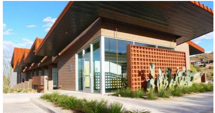
FIGURE 21—Concrete Masonry Screen Walls
