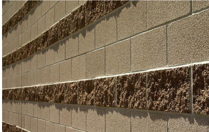
Figure 1. Using texture and color to add interest to a concrete masonry wall.
