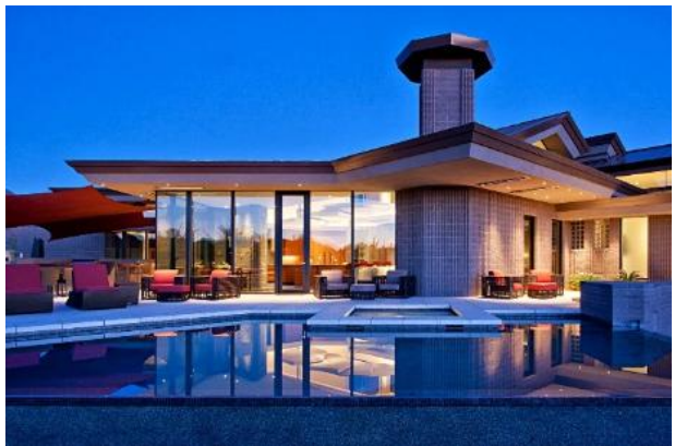
Scottsdale, AZ Architect: Swaback Architects + Planners Producer: Superlite Block Photo courtesy of Arizona Masonry Council
